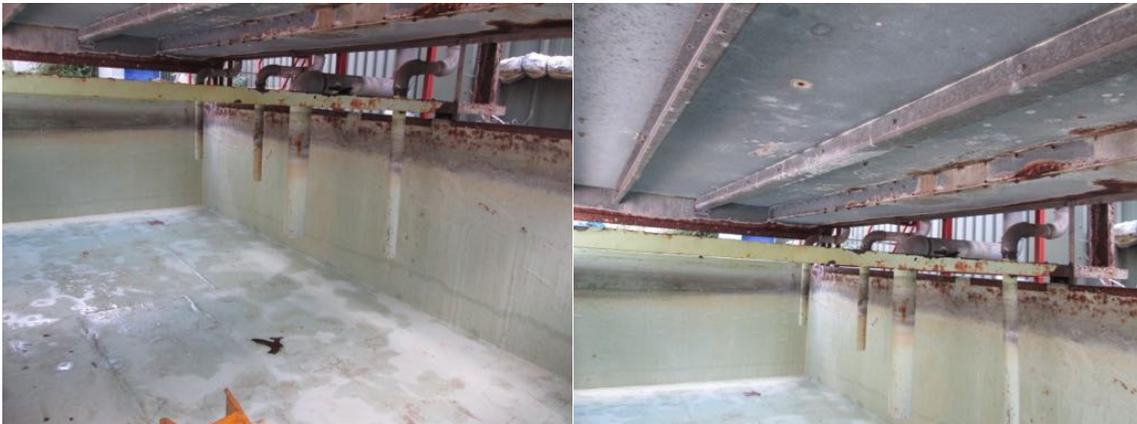
Externally, there was also signs of localized corrosion
