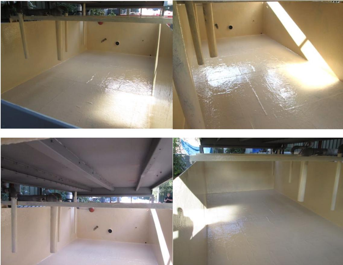
The external surfaces of the tank, and underside of the cooling tower, were then coated with a 0.5mm coat of RB MEMBRANE
