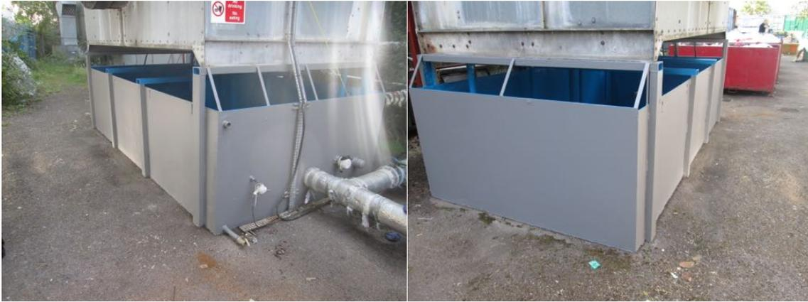
The internals were given a second coat of ACOTHANE DW applied again at a nominal thickness of 0.5mm
