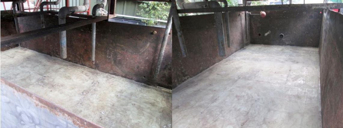
Likewise, the external surfaces were also prepared to accept the new coating.
